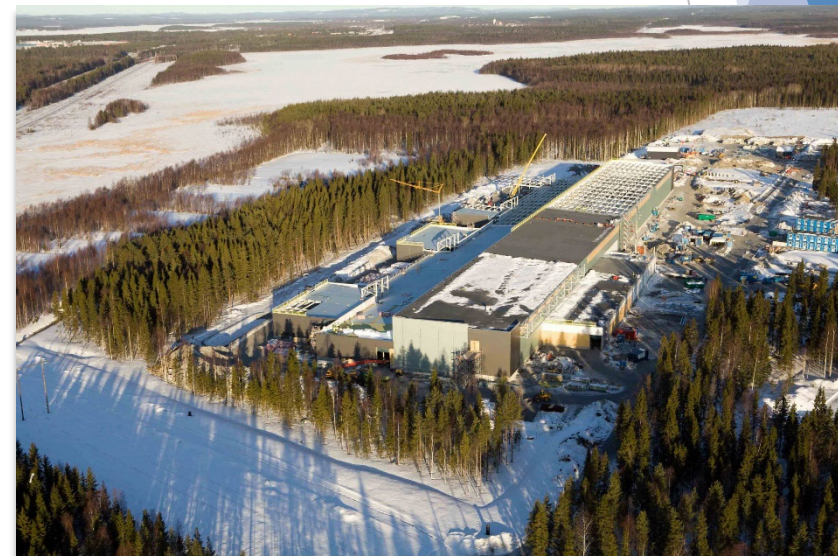
Facebook's Luleå, Sweden data center in construction in 2012. Source: Facebook
